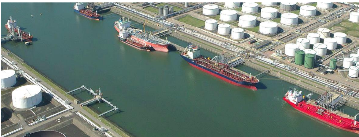
Typical mooring at sheltered berth
